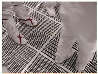
Clean air continuously flows from every pore of the ceiling and through the holes in the floor. All of the air in the clean room is replaced several times every minute.
